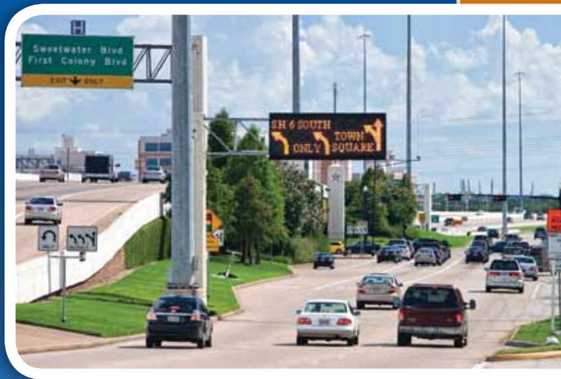
Approximately 100,000 cars per day travel through the intersection of US 59 and SH 6.
